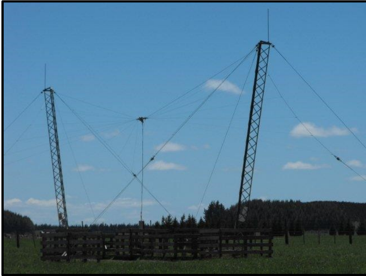
Rangitaiki Marine HF transmitting Stn 13/11/10, wide band dipole
