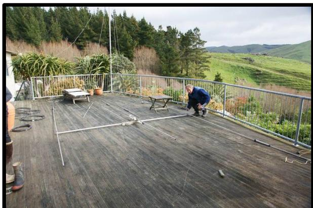
*3 element tri-band beam going together*
