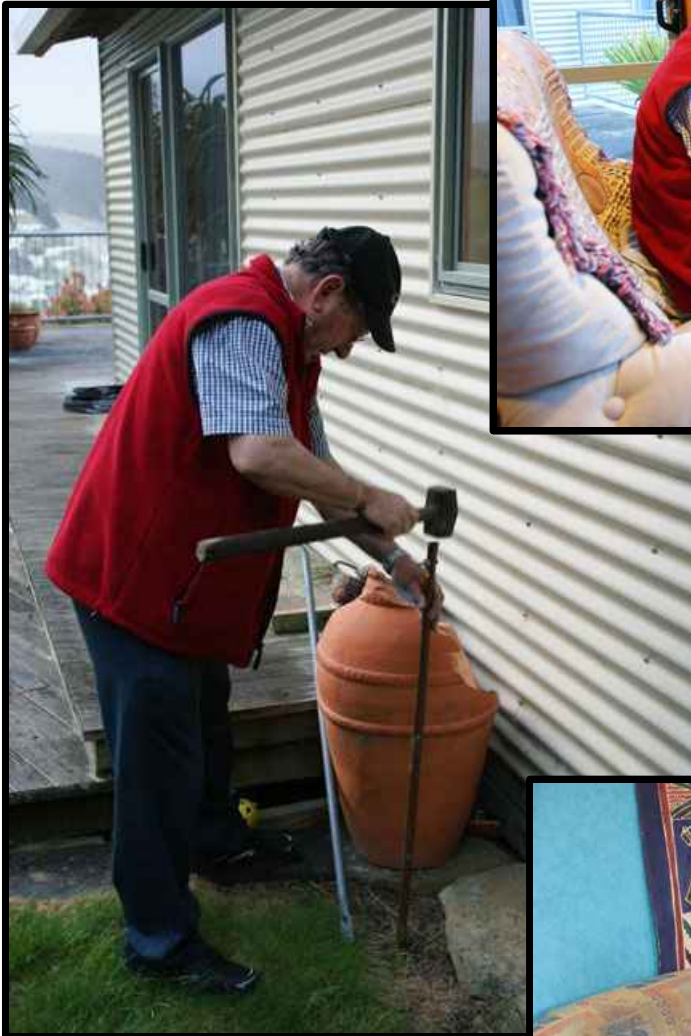
Rob ZL2US hammers in the earth stake
