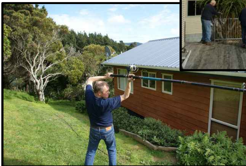
Dave ZL2OK launches an end support line for the doublet
