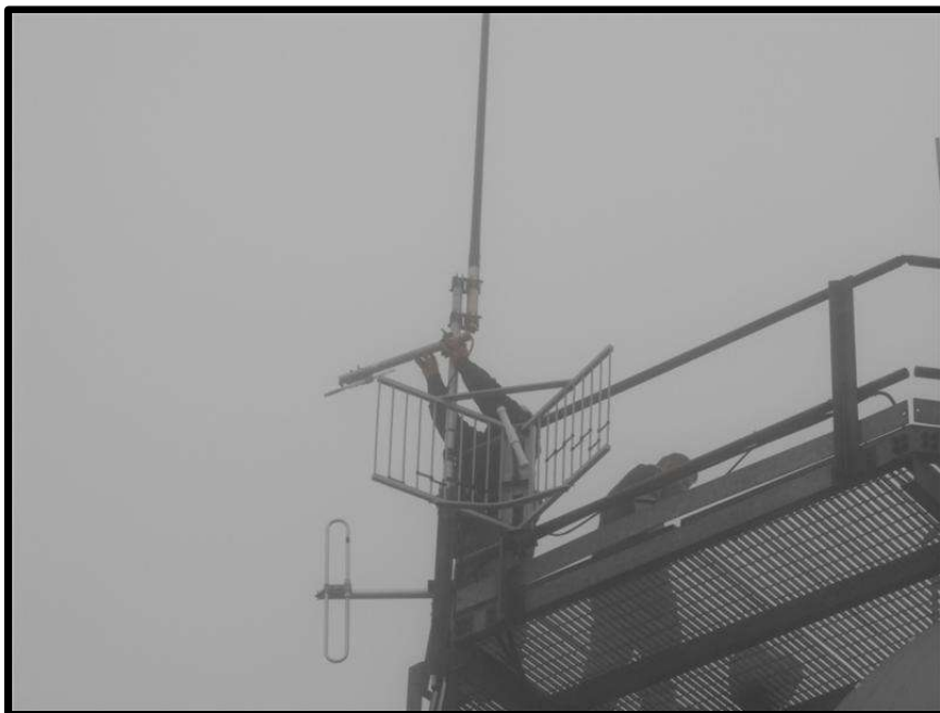
Laurie ZL2TC changing the clamp on one of the '725 aerial at Taraponui (the picture was taken from the ground and zoomed up, hence the "white" conditions as cloud swirled around)
