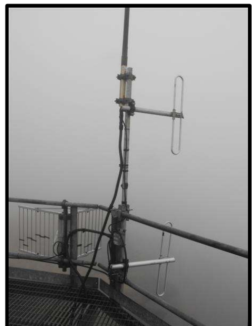
The almost finished arrangement at Taraponui. Top aerial is a UHF collinear (for '405) fed with LDF 550 coax. cable. The two phased dipoles are for the '725 repeater transmitter, again fed with LDF 550 coax. cable. (The UHF corner reflector aerial is for commercial use).
