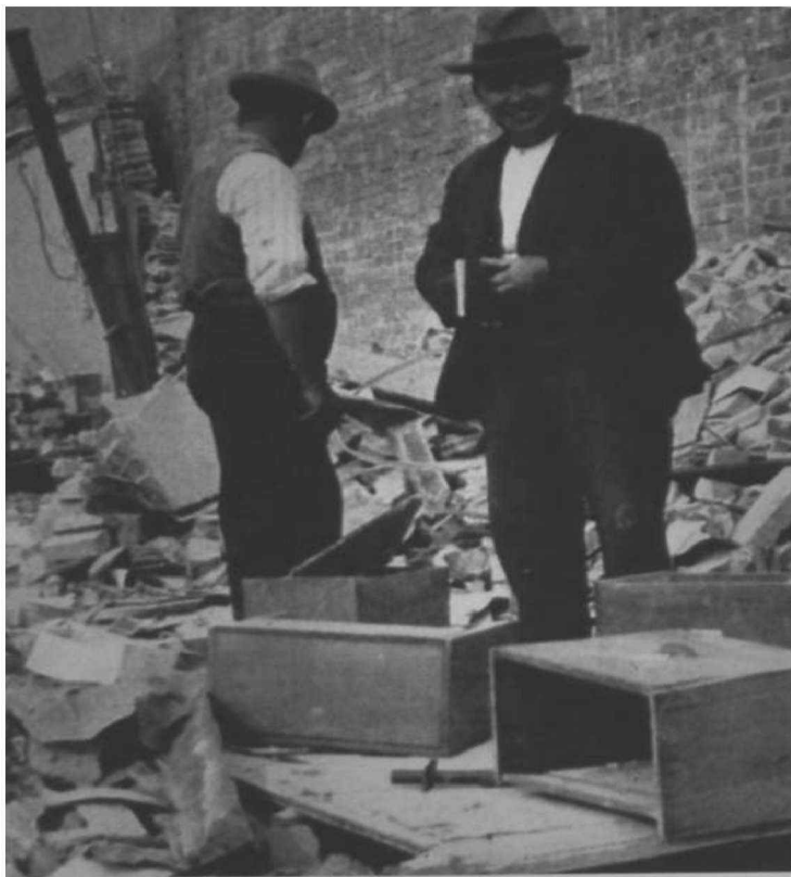
CLEANING UP AFTER THE 'QUAKE
