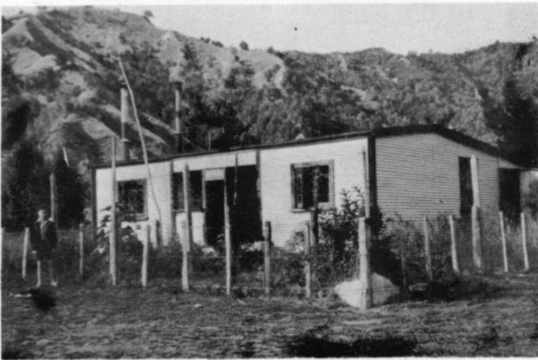
FIRST OTOI HOMESTEAD BUILT 1925
