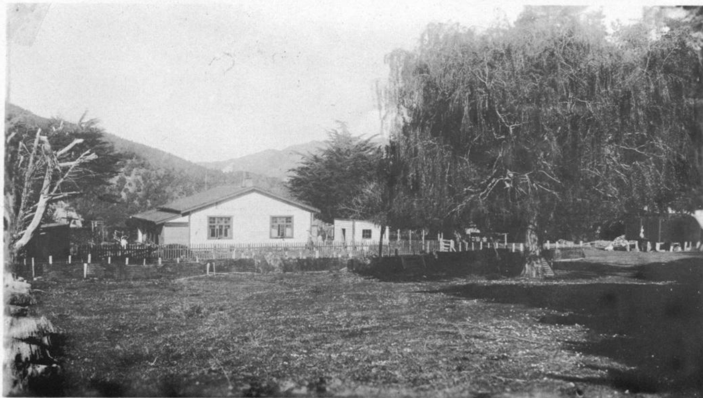
ARMSTRONG HOMESTEAD BUILT IN 1921—22 BY JIM GRANT AND JACK THOMPSON. DEMOLISHED IN 1975
