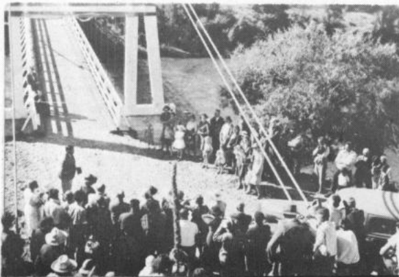
OPENING OF OTOI BRIDGE, 1940
