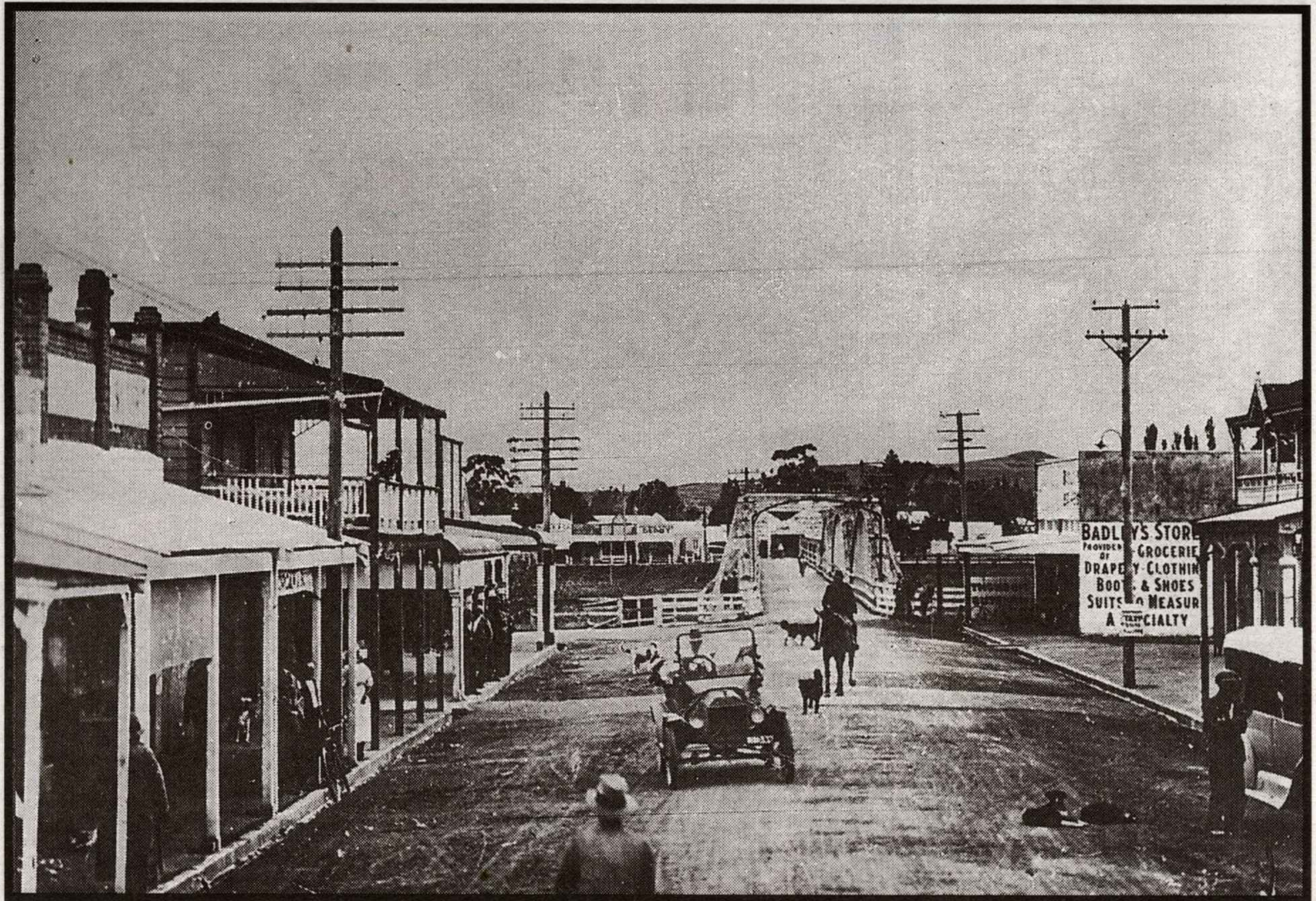
A view from North Clyde of the old Wairoa traffic bridge, which replaced the ferry as the horse gave way to the car.
