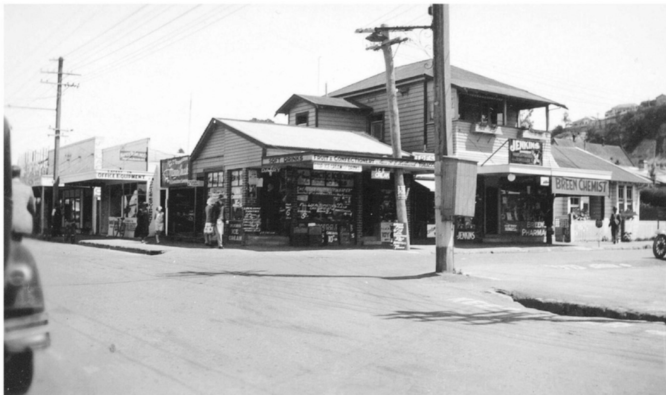
To the right of the photograph can be seen the signs BREEN - CHEMIST and JENKINS - JEWELLWER. The two storeyed building, which was No.5 Clive Square West, was shared by Breen & Jenkins for a few weeks after the 'quake.
