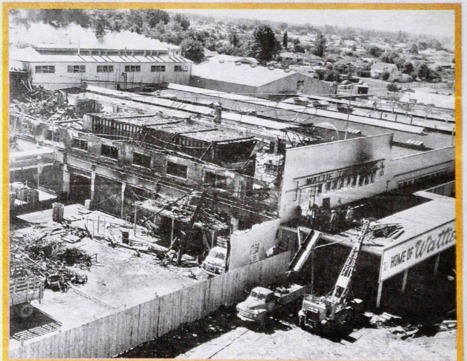
BELOW: 1962 fire devastated J. Wattie Canneries Ltd in Hastings.
