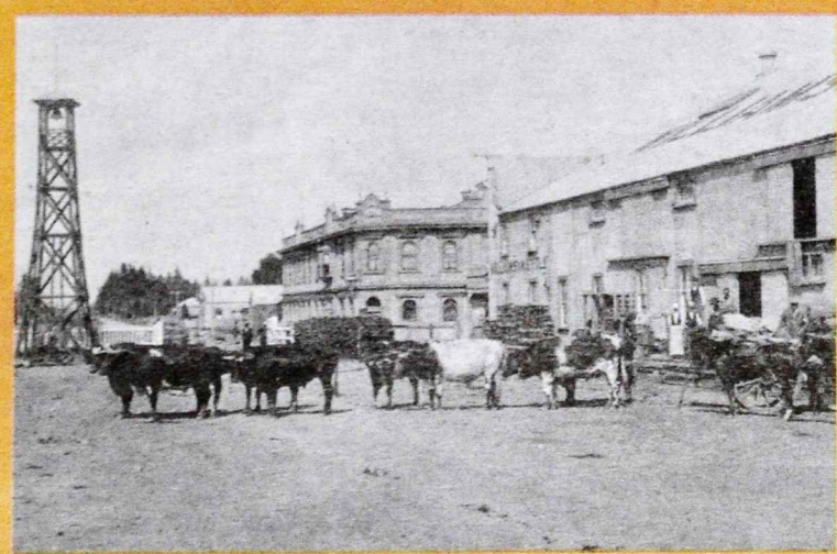
ABOVE: Williams & Kettle Ltd's Railway siding - note the bullock team.
