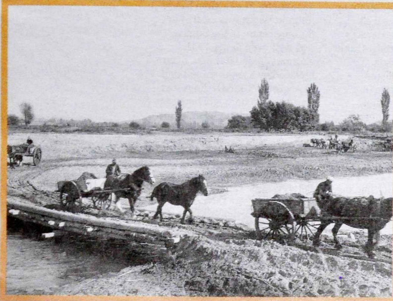
Flood control work started as early as 1877 and stopbank construction and maintenance has been essential to protect the plains from frequent flooding
