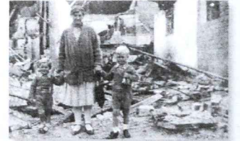
David, Rita & Syd Taylor in the remains of the Taylor's building, Emerson St after the 1931 earthquake
