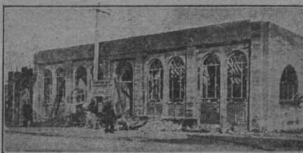
One of our New Building Contracts in the Course of Erection.
