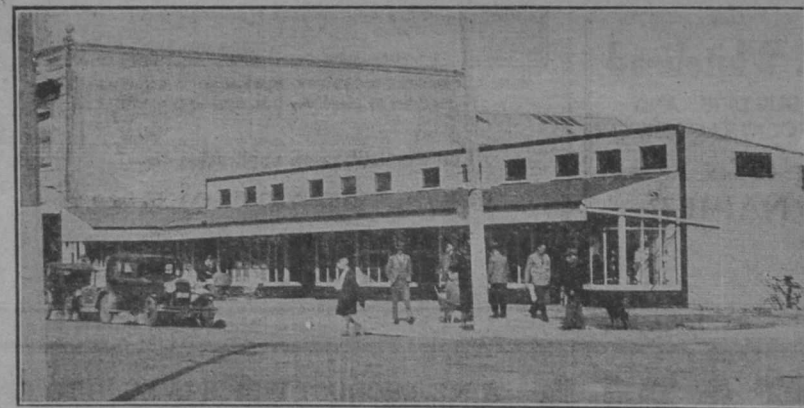
Replacing a familiar landmark. Messrs. Roach's temporary premises, Hastings, erected on the site of their wrecked department stores.
