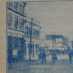
During the trying days of the first week in February, the people of Napier and Hastings learned to walk in the middle of the road to avoid falling debris. This habit still persists to some extent, as can be seen by the above, a recent scene in one of the less severely damaged streets of Napier.
