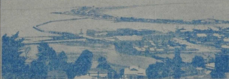
Port Ahuriri, Napier, was damaged to a very considerable extent by the raising of the sea bottom. In the above photographs mud banks, many acres in extent can be seen where fairly deep water was previously found.
