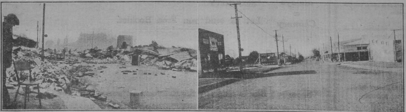
Hastings after the earthquake and to-day. The above views afford an excellent idea of the reconstruction work that has been carried out since February 3.
