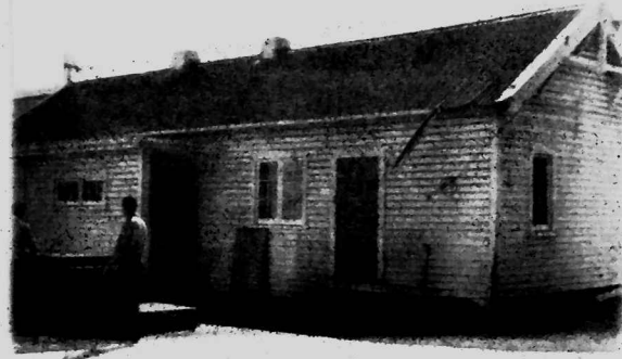
The building where industrialist Sir James Wattie set up his food processing plant in 1934.
