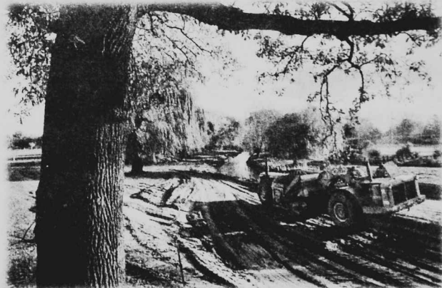
IN 1985, Withers earthmoving machinery widened and deepened the creek at Fantasyland to accommodate the paddlesteamer.
