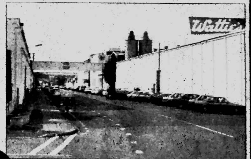
The King Street Factory as it is today.
