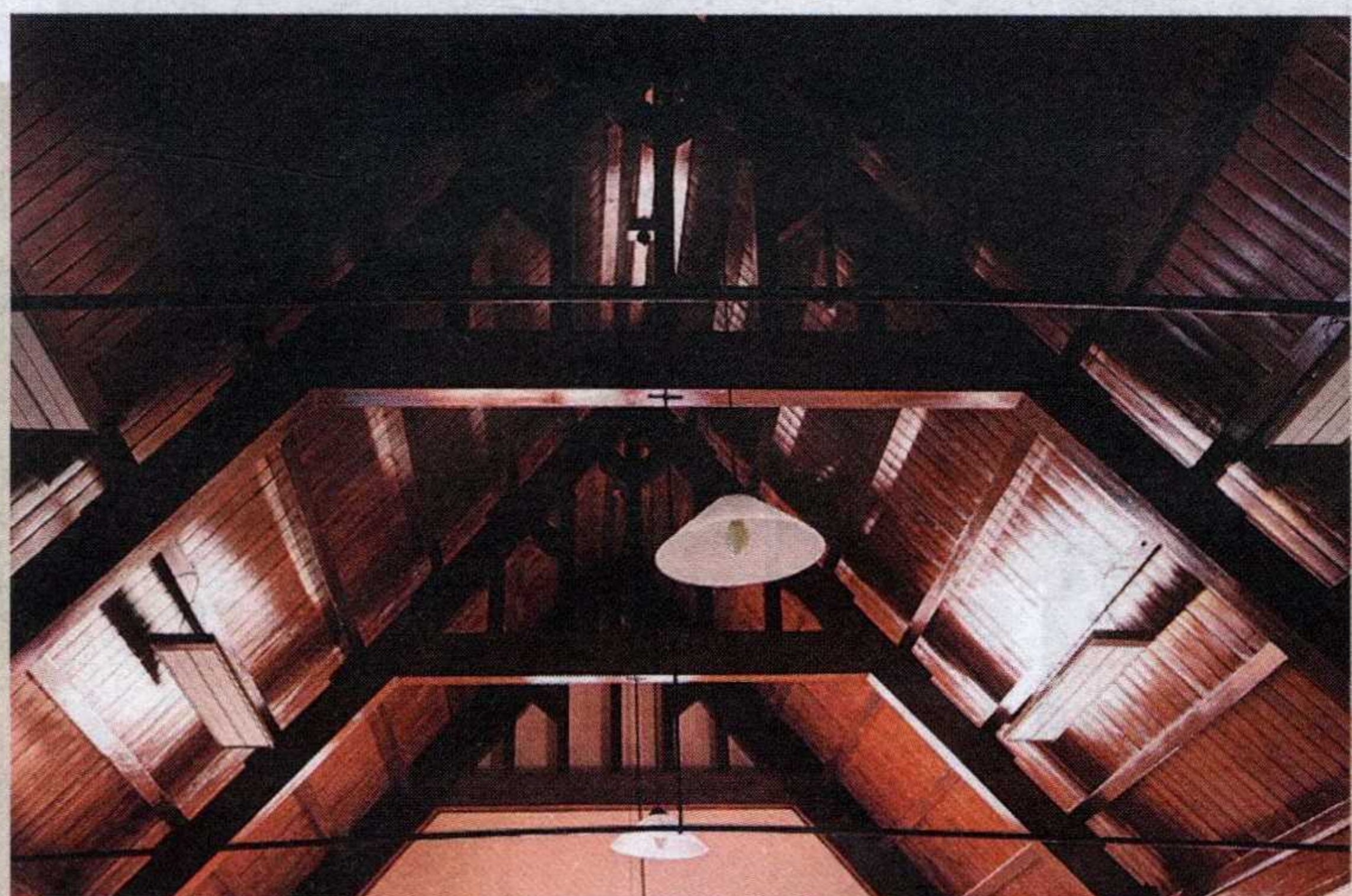
ABOVE: St Georges Chapel, Interior ceiling after the renovations.
