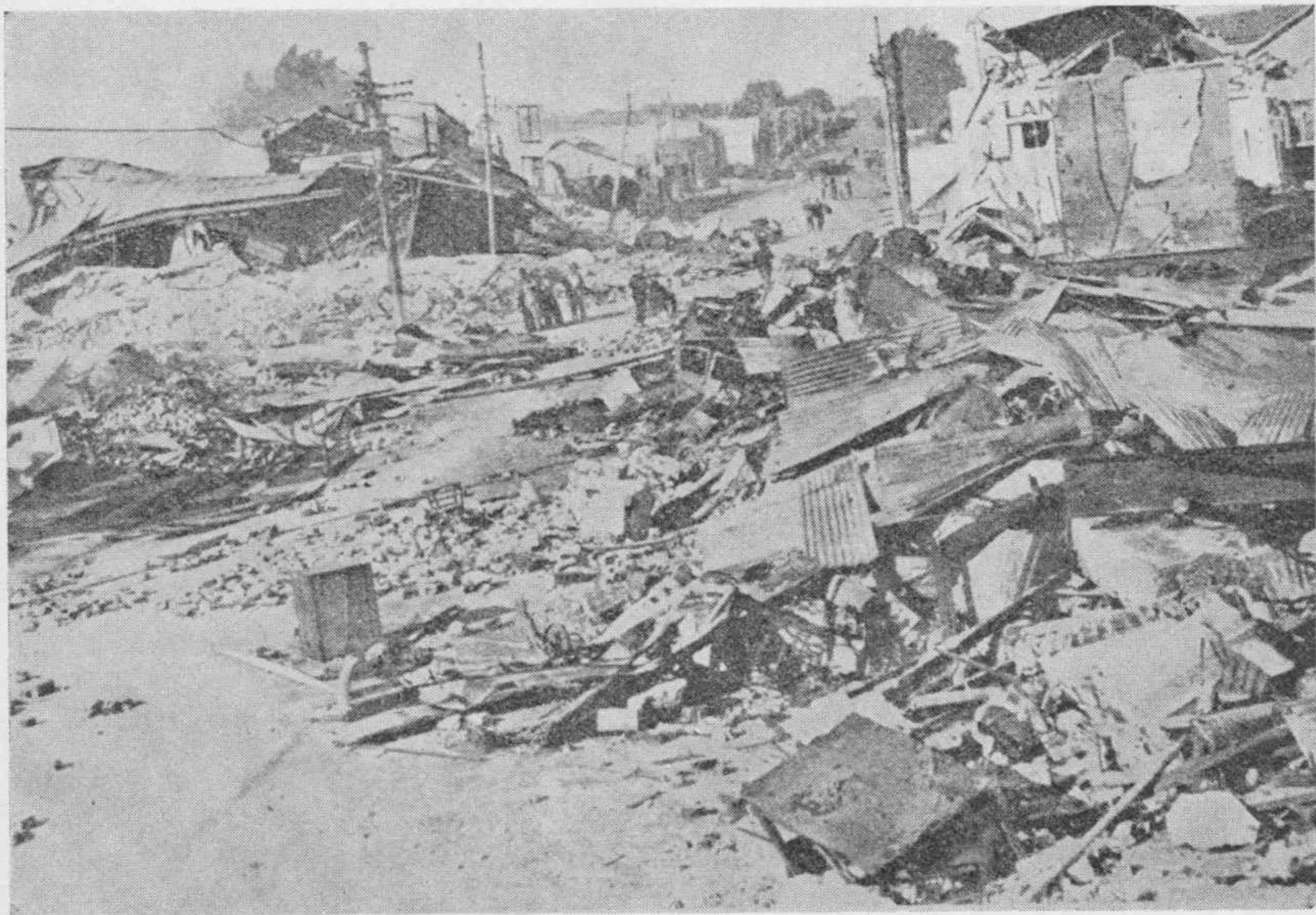
FIG. 7.—Street scene in Hastings after the earthquake.
