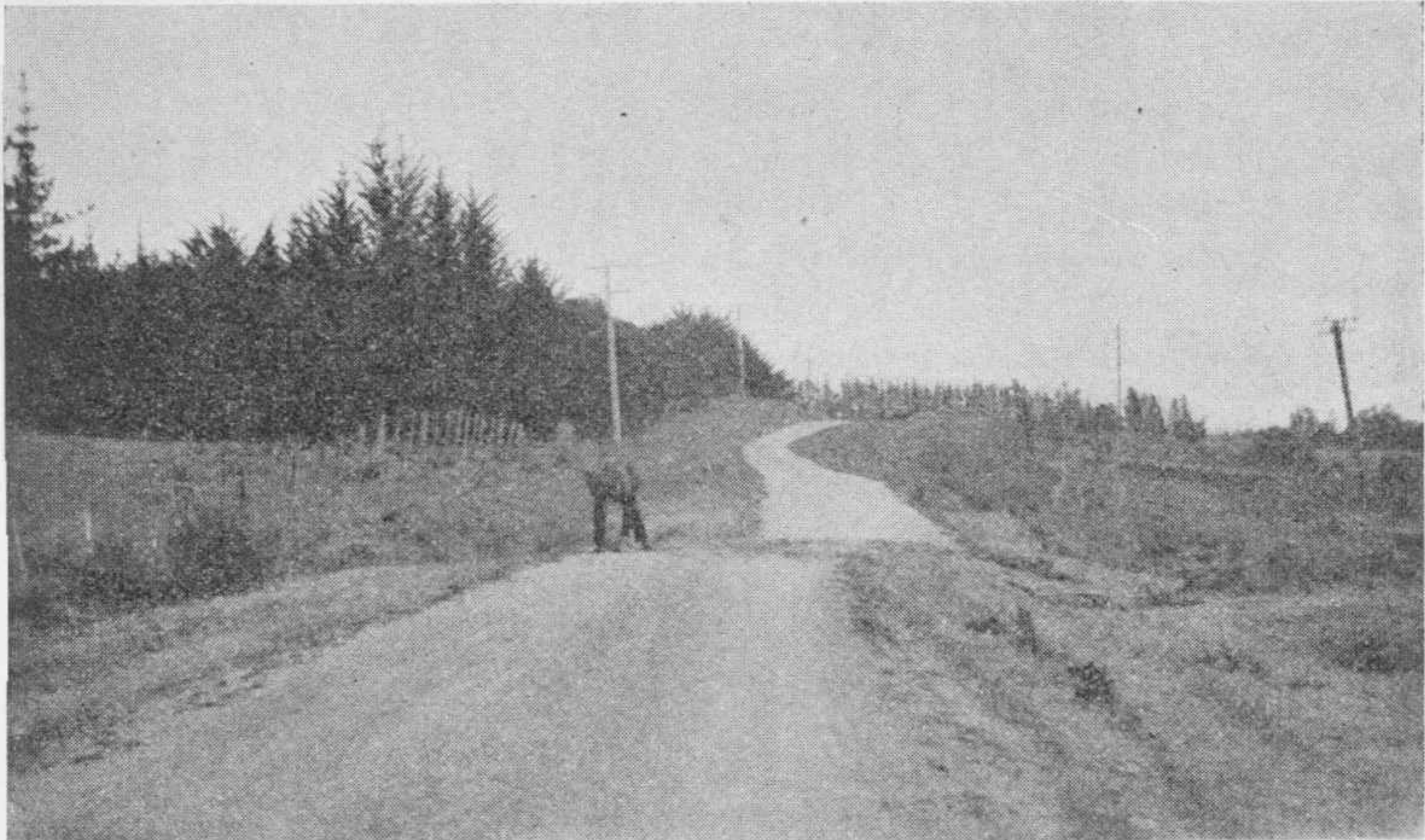
PLATE VII.—( a ) Road east side of railway, two and a half miles north-east of Poukawa Railway-station. The displacement is between 6 ft. and 7 ft.
