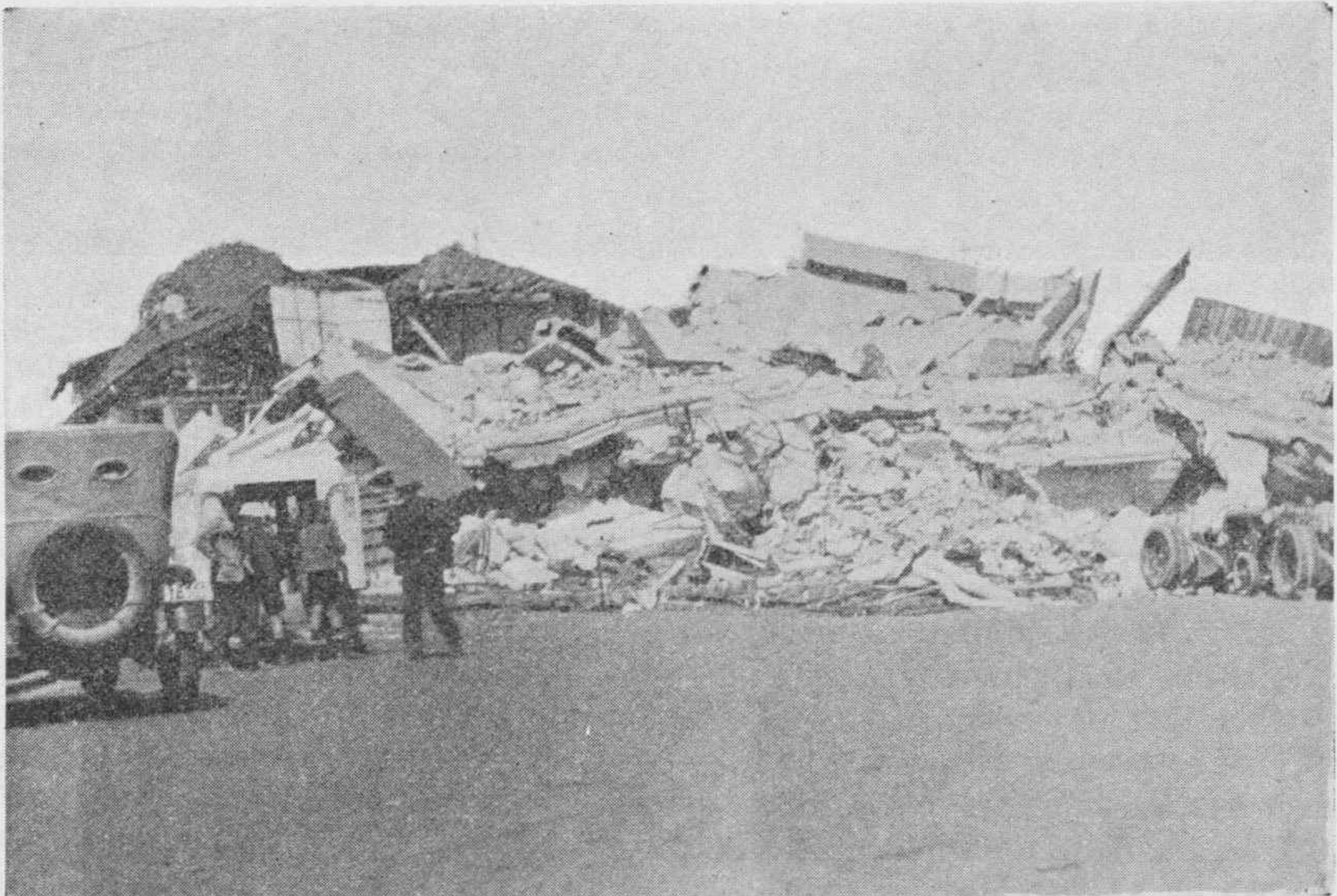
FIG. 4.—Nurses' Home, Napier Hospital, immediately after the earthquake, taken from approximately the same position as fig. 3.
