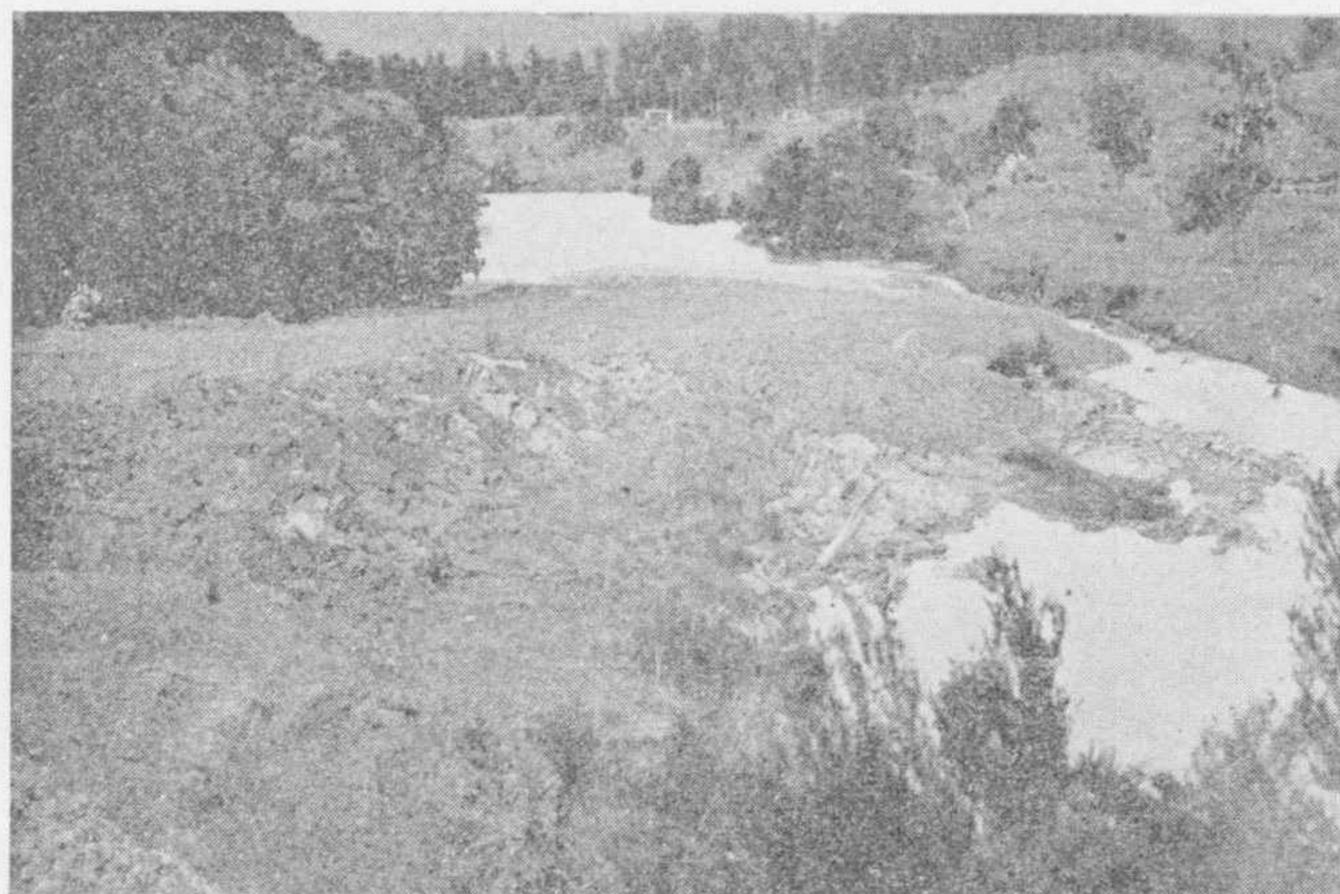
FIG. 3.—Mud blowout on Mr. J. Barnes-Graham's property blocking the Hangaroa River.
