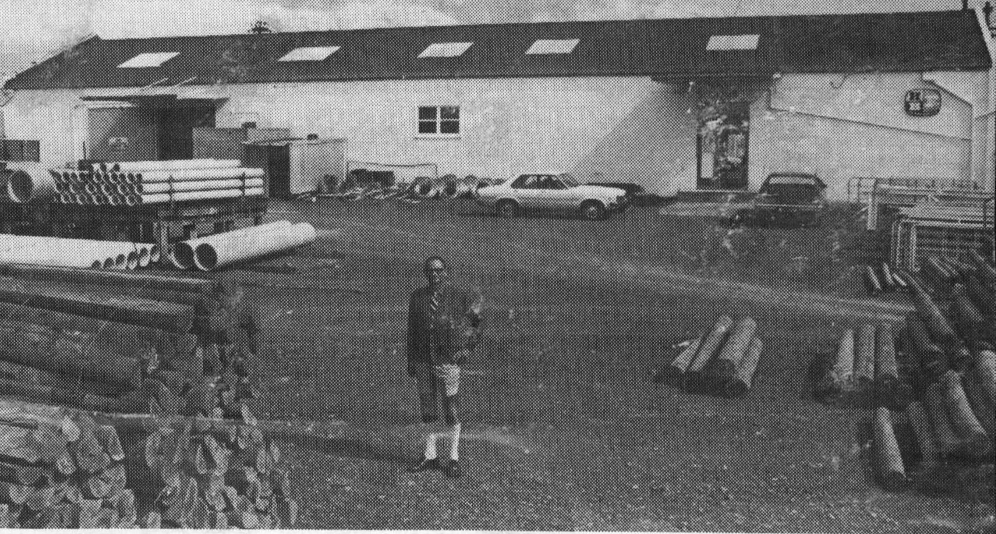
What is now the produce store — shown here behind Ian Wilkinson, produce store supervisor — originally housed the entire HBF operation in Dannevirke. HBF does a brisk business in stock feed. Another best-seller is Fibrolite pipes (shown left centre) for which HBF is sole agent in Dannevirke. A 400-cubic-foot refrigerator stores Total Dog Food, another product for which the company is sole agent there.
