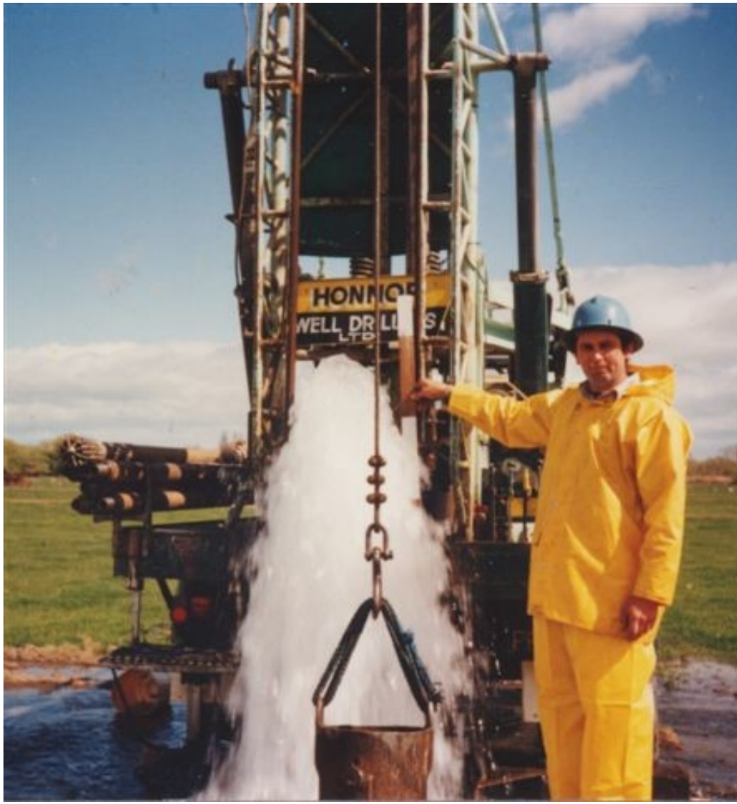
Paul Bower's pride, Farndon Rd., Sept. 1987. --- (And record free-flow of 84,000 GPH from 6" well still remains 2009).
