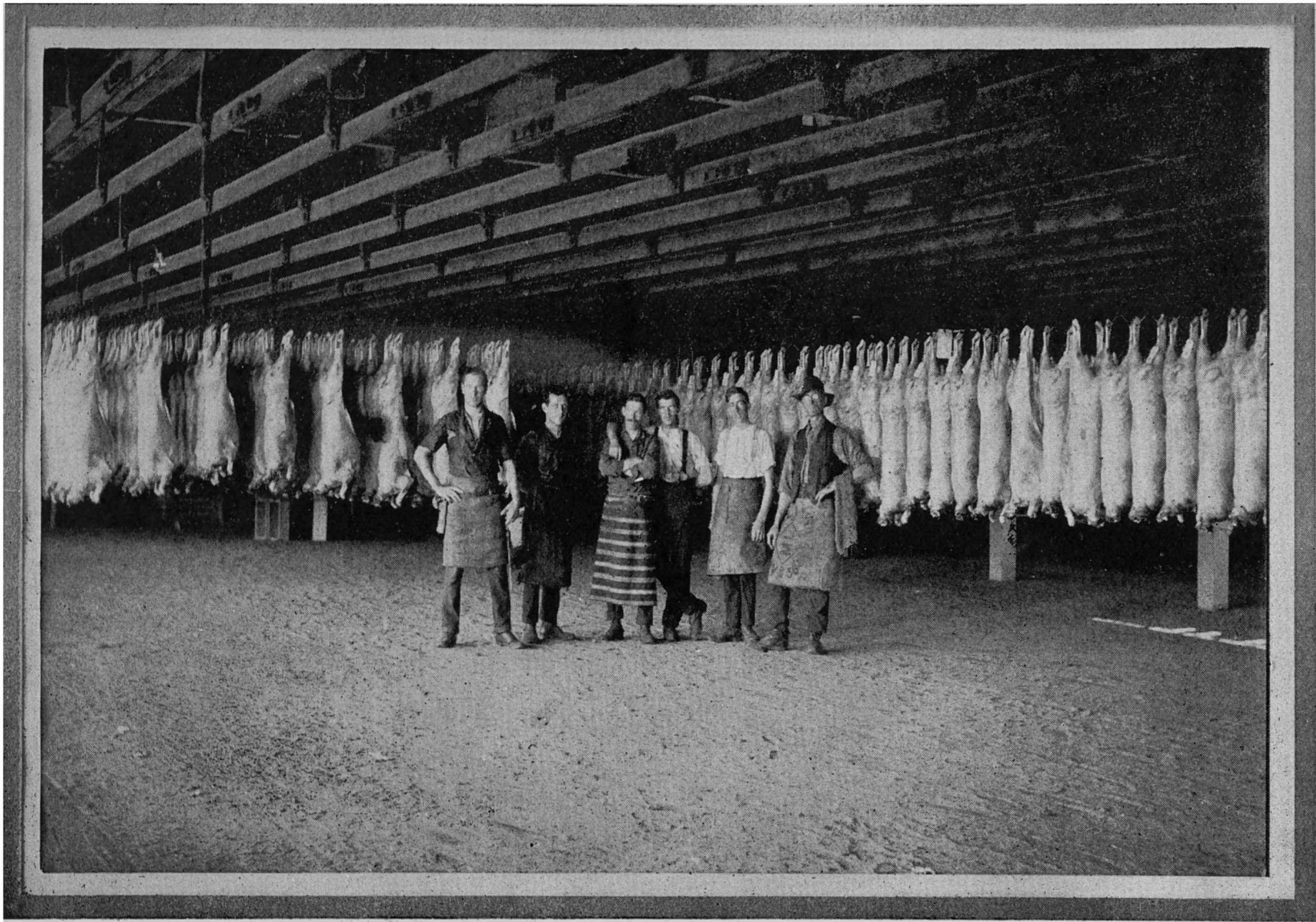
The Cooling Room
