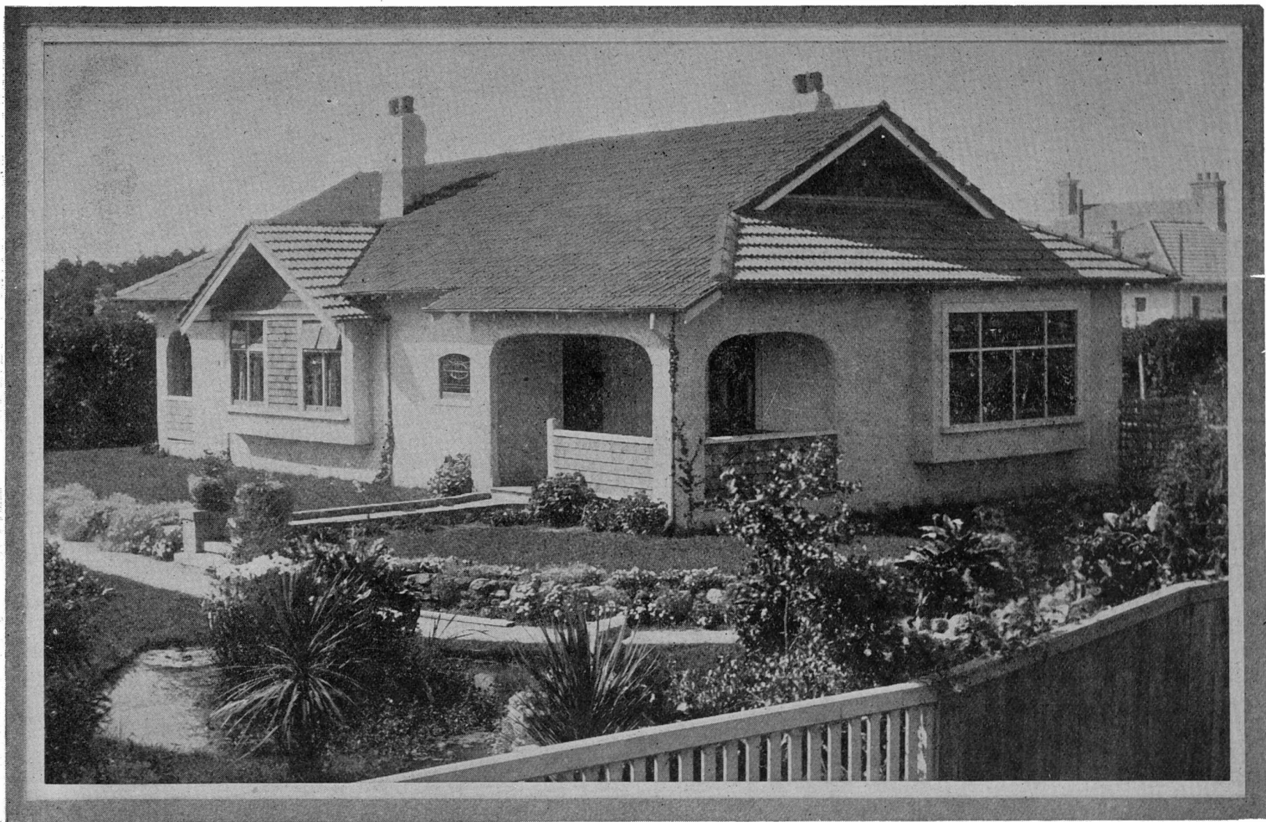
“Roycroft”—A Suburban Bungalow, Hastings.
