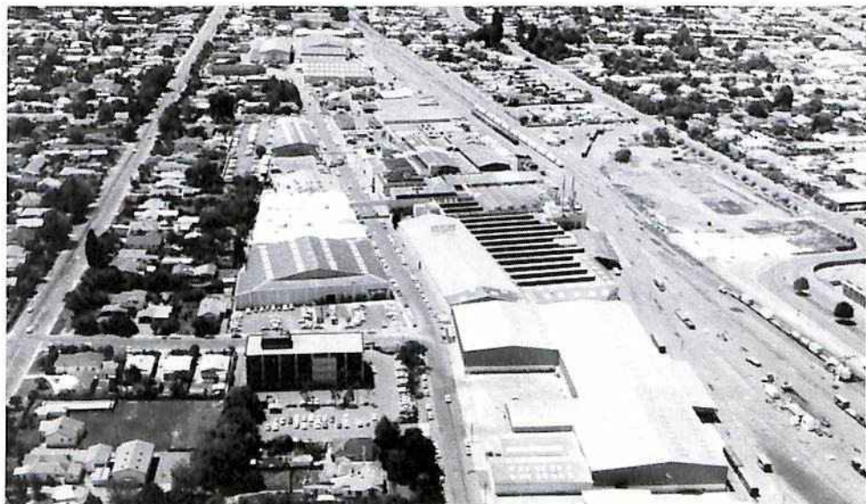
Hastings Factory site today
