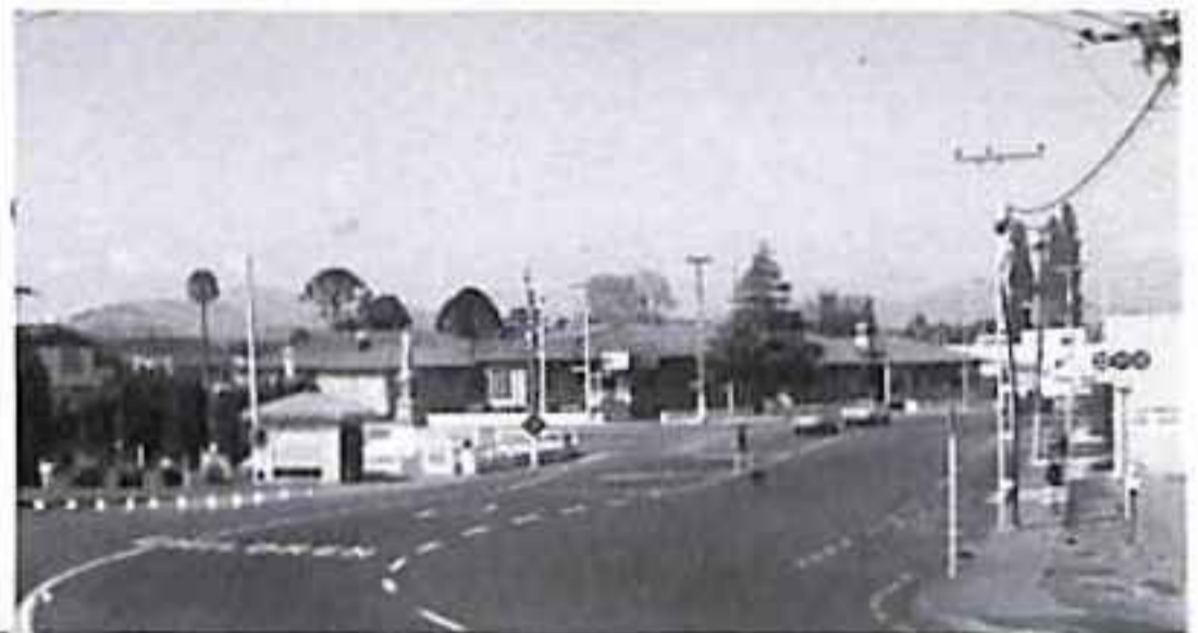
Above:— Clive Township looking south;
