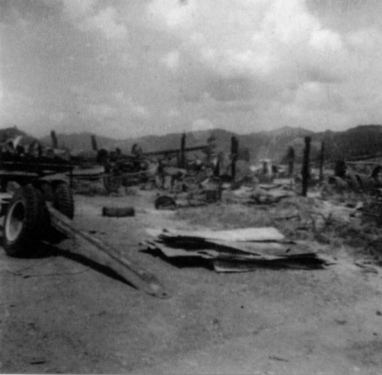
Odlin Timber & Hardware Ltd, - sawmill, Pohokura. Napier Taupo Road. - The burnt out sawmill. Photo : cleaning up 17 th February 1964.
