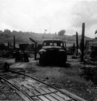
Odlin Timber & Hardware Ltd, - sawmill, Pohokura. Napier Taupo Road. - Burnt out Austin sawdust / slab truck was parked inside the sawmill building. Photo ; cleaning up 17 th February 1964.
