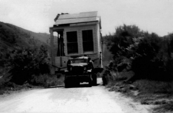
Tuck Bros Ltd , sawmill, Tataraaikina Timber Co, Tarawera, HB. - GMC logging truck carting section Tarawera School along Napier Taupo Road to new site on sawmill grounds. : Photo Christmas holidays 1951.
