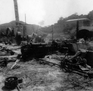
Odlin Timber & Hardware Ltd, - sawmill, Pohokura. Napier Taupo Road. Foreground, all that's left of the breast bench saw after the fire. Photo 17 th February 1964.
