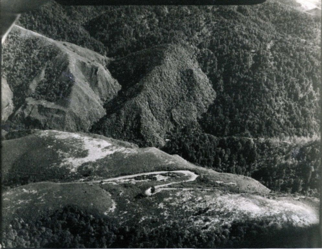
Runanga section between Tarawera and Pohokura.- hair pin bend on the Napier Taupo Road. New road follows the Waipunga Valley just below this steep hill. : Aerial photo. 2 nd September 1949.
