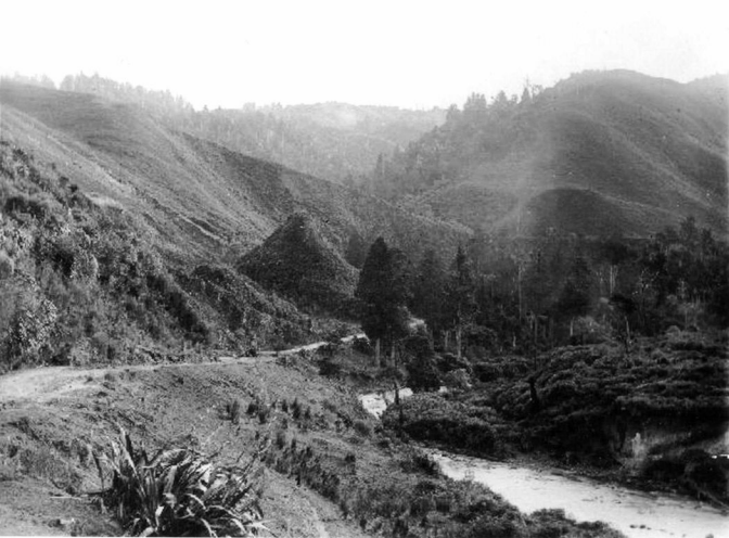
Napier Taupo Road - over the Tarawera saddle, Taupo side of Tarawera, the Nunnery area. The river is the Waipunga. Photo : September 1896.
