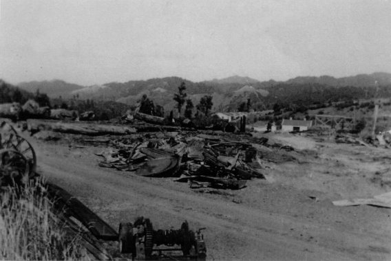
Odlin Timber & Hardware Ltd, - sawmill, Pohokura. Napier Taupo Road. Burnt out sawmill machinery reduced to scrap metal. : Photo 17 th February 1964.
