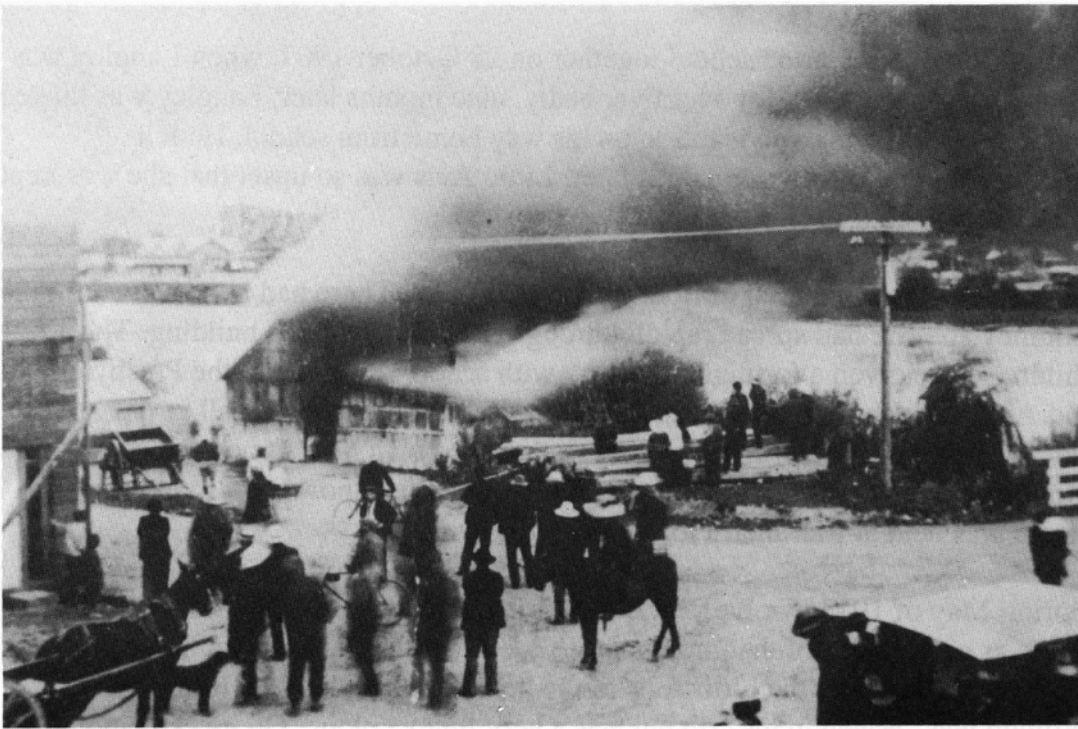
Fire at HW Brown's Shop
