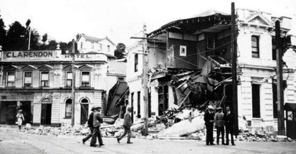
Hawke's Bay, New Zealand, Earthquake February 3, 1931. Earthq...
