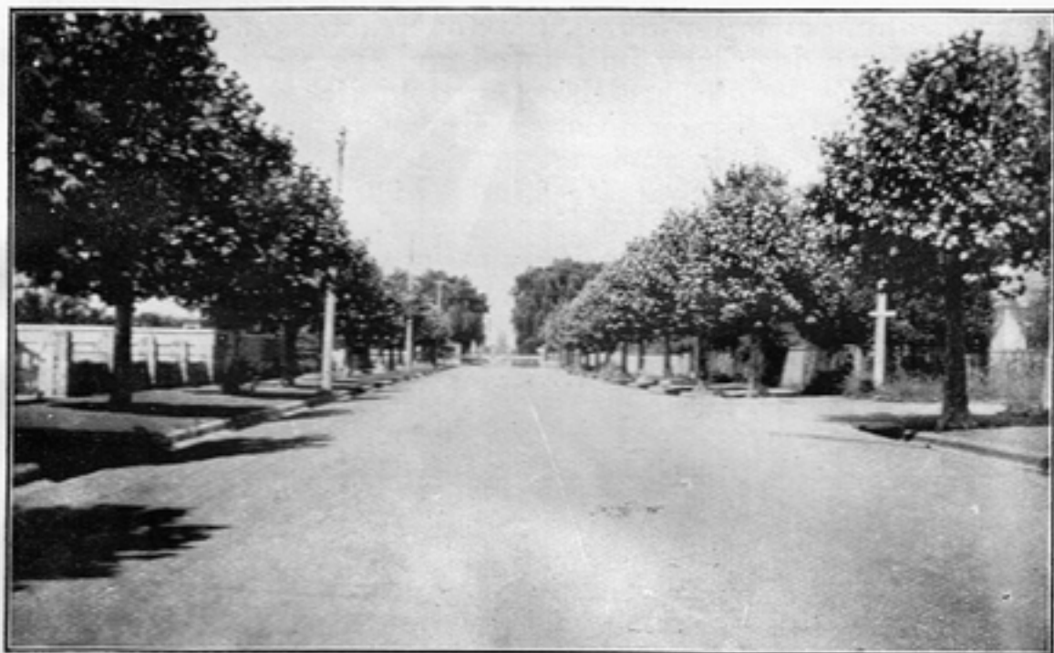
Market Street, Racecourse Entrance.
