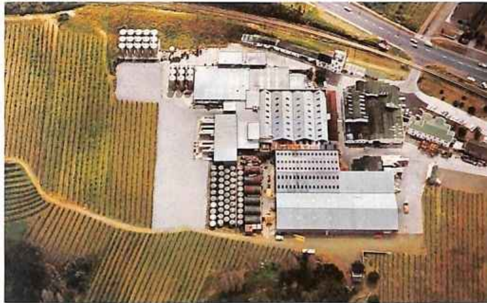
Corbans Henderson Winery is set in the original vineyards.
