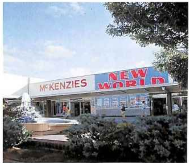
Modern commercial property in Otara's Town Centre.
