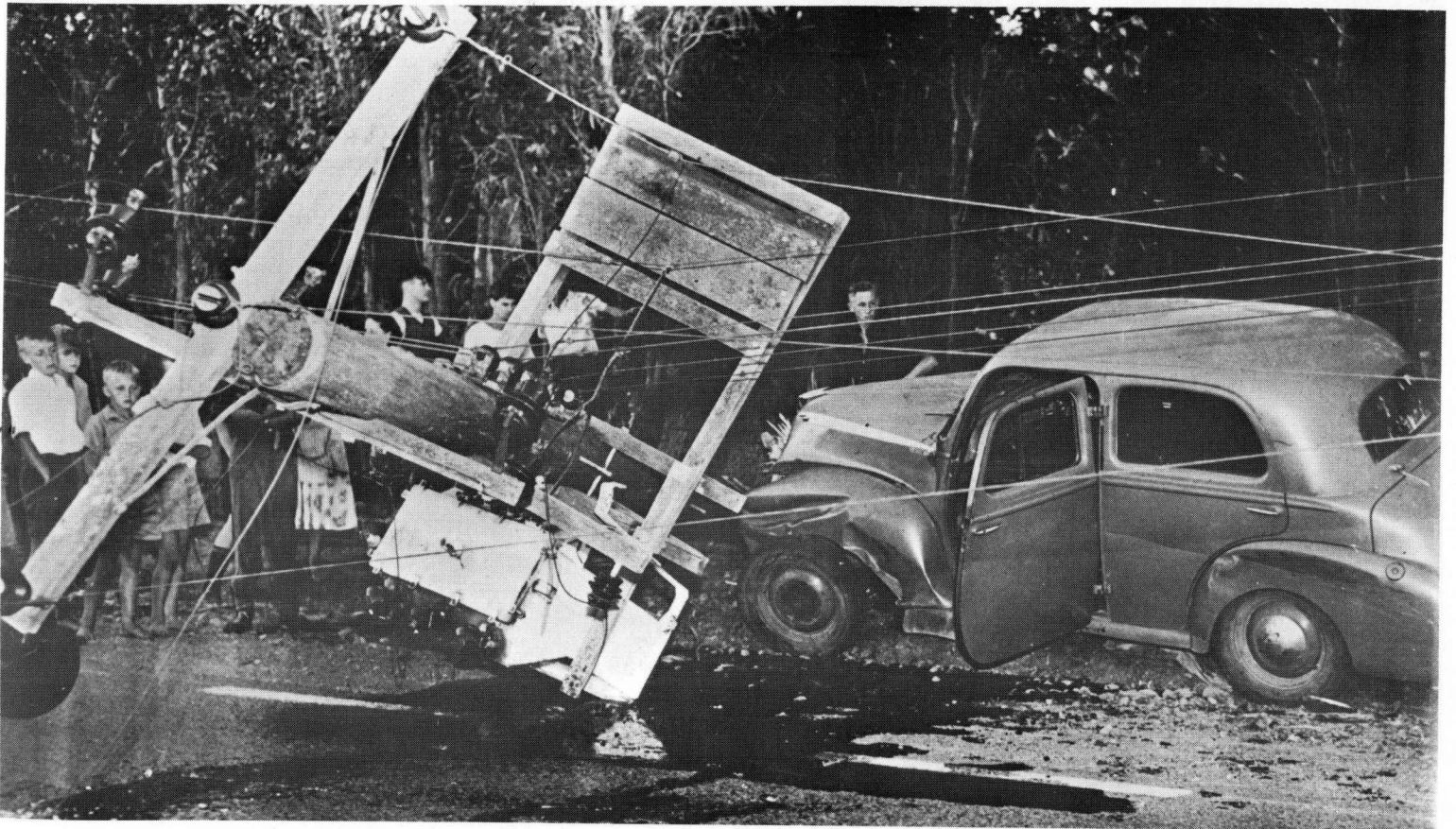
When a motor vehicle travelling at speed encounters a solid powerpole results can be spectacular and troublesome. This car crashing into a pole carrying two sets of lines and a transformer in Omaha Road, spelled trouble for all concerned. The crash dropped 11,000-volt lines on to 230-volt circuits. Many people had a cold tea in the district that night.
