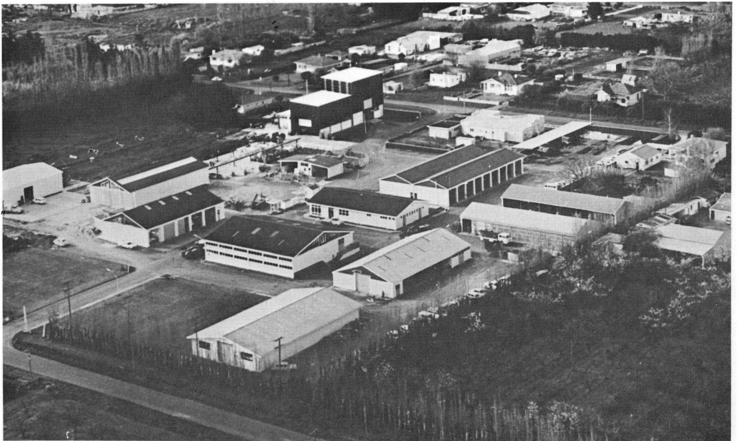
Acquisition of the appropriate land and development of the Howard Street depot were vital steps in the growth of the board. Situated on the eastern side of Hastings city, the large depot serves a multitude of purposes.
