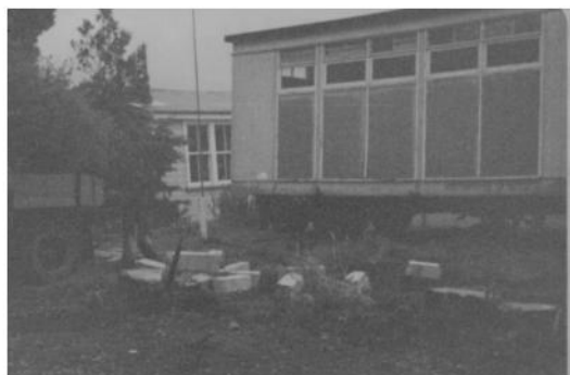
Moving in the replacement room
