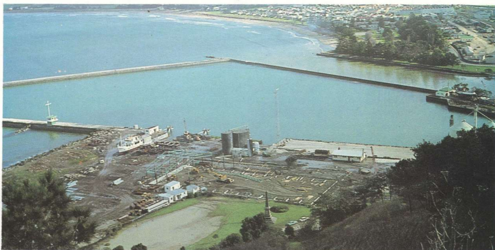
Looking down from Kaiti Hill on the new cold store.
