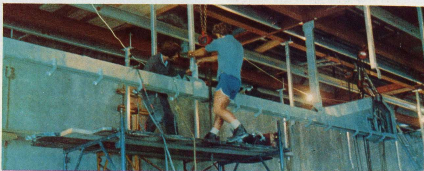
Installing one of the three chains on the dressing floor.
