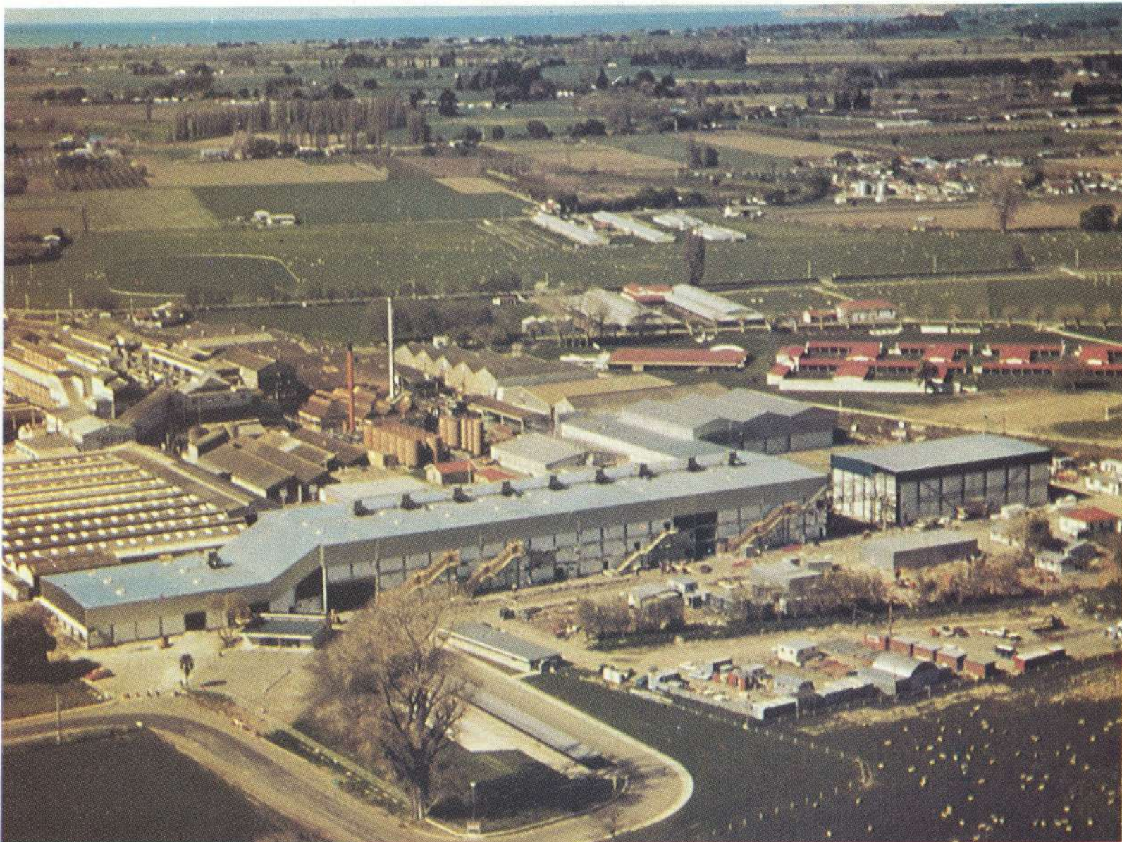
The new mutton complex dominates the Tomoana scene as it nears completion. From left the complex is made up of the stockyards, three storey slaughterhouse, with the freezing chamber at the right and cool store and rail loading siding at the rear.
