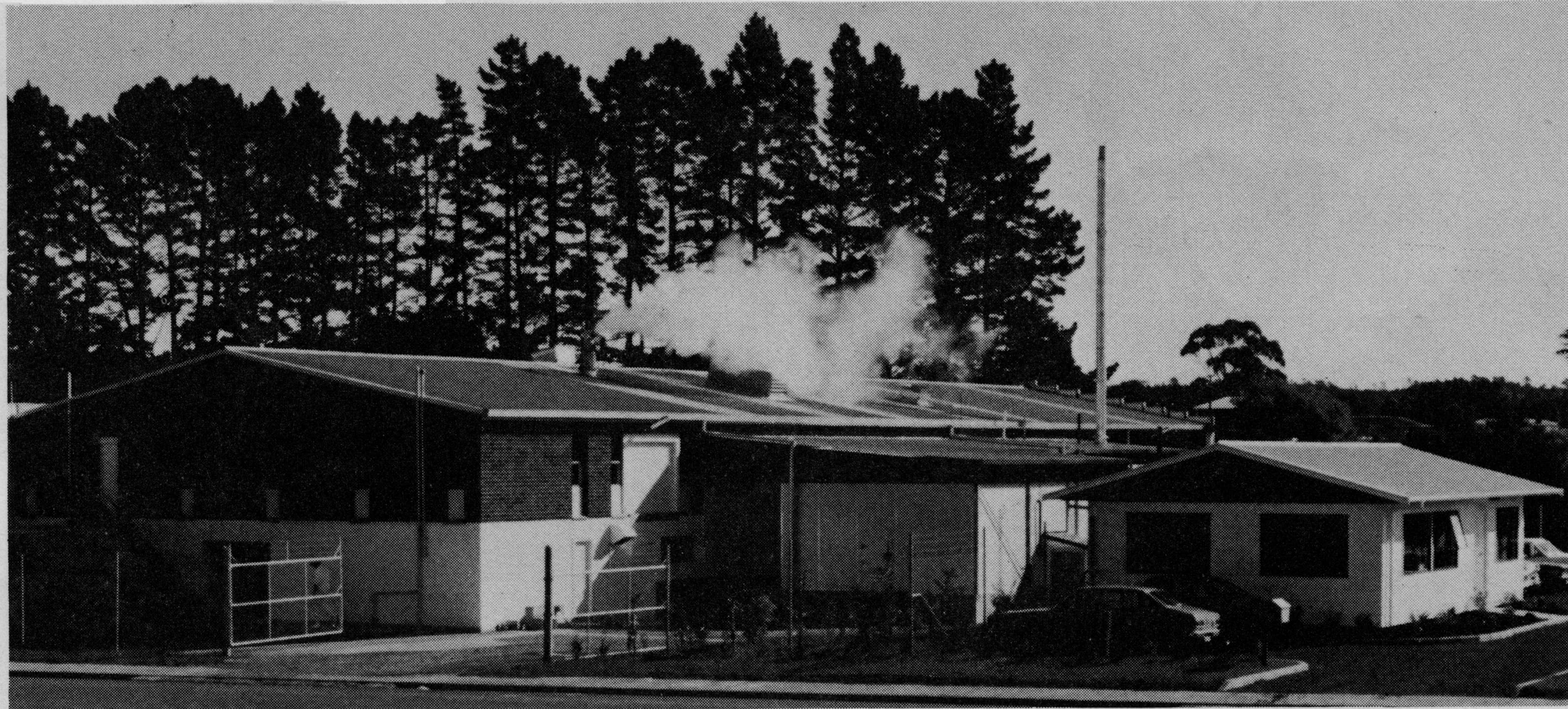
THE smart new premises at Henderson, Auckland, provide a sharp contrast and a vast improvement on the previous cramped factory at Waitakere.
