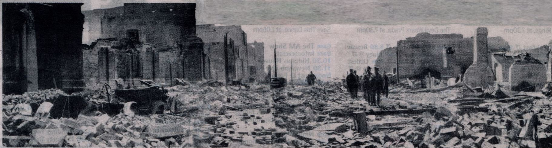
In 1931, a 7.8 magnitude earthquake struck Hawke's Bay, killing 247 people and badly damaging or destroying buildings along the east coast.
