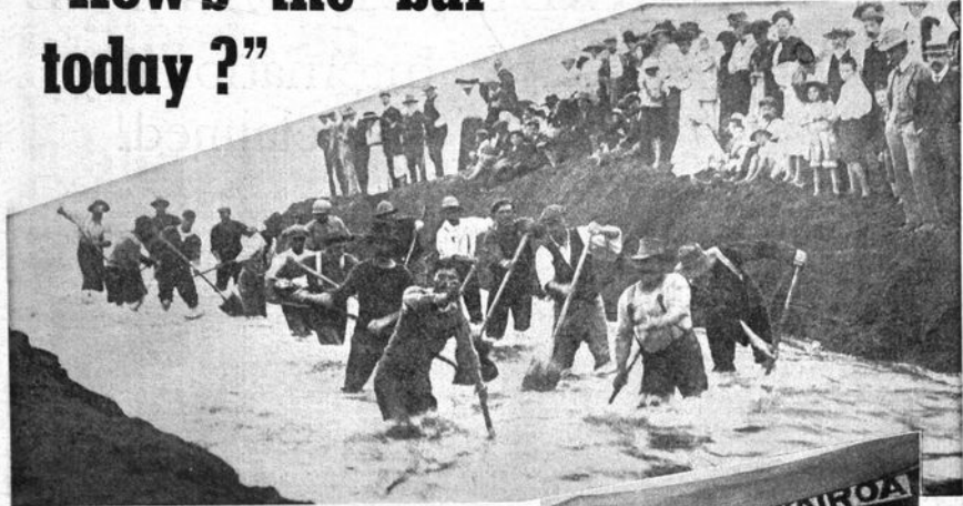
● Shovels and manpower open the Wairoa River bar in 1911. The state of the bar, which often cut Wairoa's steamer contact with the outside world, was of daily concern till the advent of adequate road and rail links.
