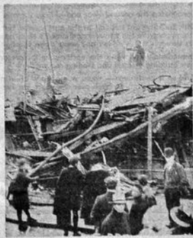
Smoking ruins of the Gaiety Theatre, Napier, destroyed by fire on June 6, 1911. The theatre was re-opened on a section opposite, in Dickens Street.
