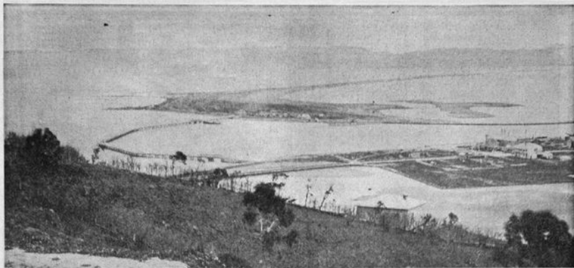
▲ Ahuriri almost a century ago. The lagoon stretches to the hills, over the site of the present Hawke's Bay Airport. At right can be seen the masts of sailing vessels and the old Ahuriri Hotel (extreme right) situated on the site of the present Rothmans Tobacco Co. factory. The Westshore bridge (left) ended the ferry era.
