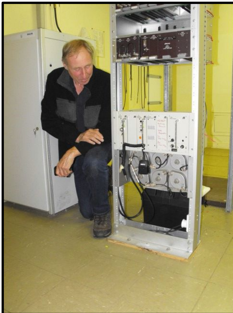
Errol Lilley (ZL2IT) beside the '670 repeater. "His" aerial filter(s) can be seen at the bottom of the rack – more in the "Living History" Article inside
