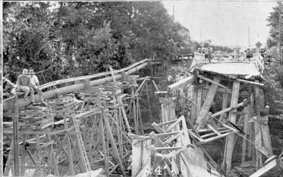
2. Havelock Bridge before the 'quakes of 9 p.m. on 3/2/31. —Photo., French Series. 4. Havelock Bridge after 9 p.m. on 3/2/31. The bridge has been totally demolished. —Lovell Smith, photo. Page Seventeen
