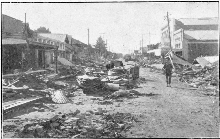
Some of the damage in third block, Heretaunga Street West.
