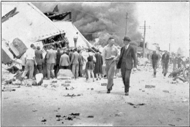
Immediately after the 'quake fire raged in the ruins of Roach's big departmental store. This photo was taken while rescue work was proceeding.
