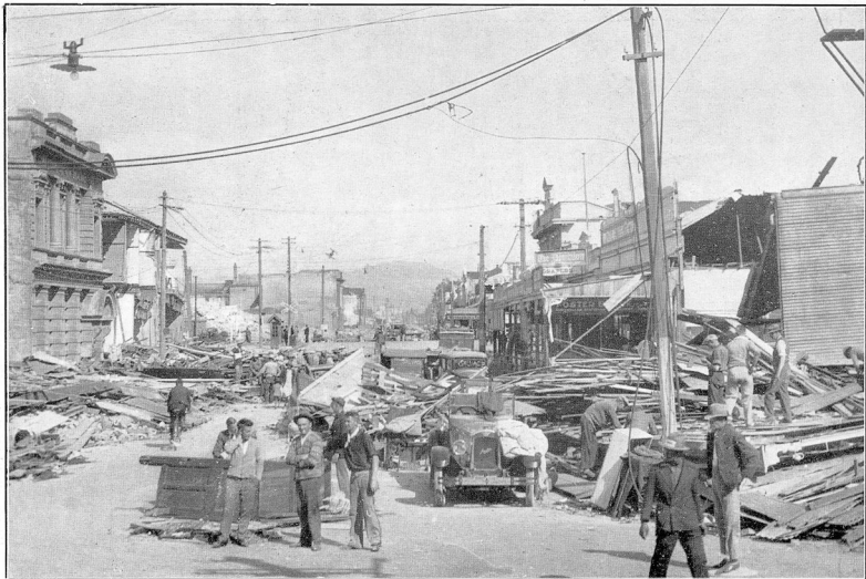
FIRST BLOCK, HERETAUNGA STREET WEST. Bank of New Zealand on left, which had to be demolished. Picket on guard in centre.
