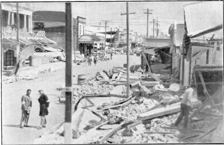
Some of the damage in the third block in East Heretaunga Street. On the right are ruins of Spencer's Garage, not out of builder's hands.
