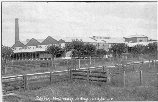
Each of our three meat works suffered extensive damage. The greatest destruction was at the Paki Paki works. This picture shows the works before. —Photo, French Series.
