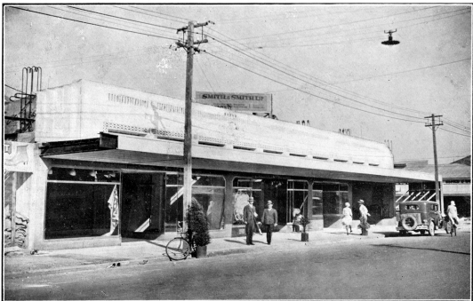
Part of restoration work in third block, HERETAUNGA STREET WEST. A new, handsome, Cosy Theatre will be built on the location of the one destroyed.
