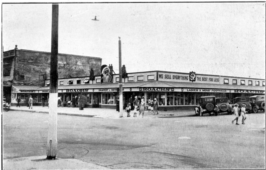
Risen from complete ruin, Roachs' new store on old site.
