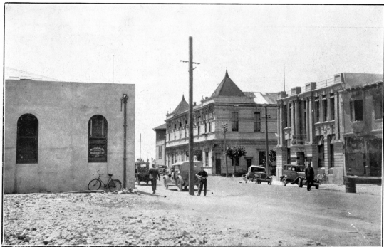
The same locality as above now restored.
