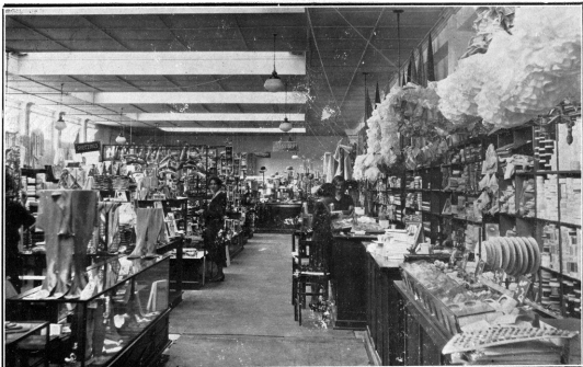
Restoration work and improvements at Baird's now complete.
