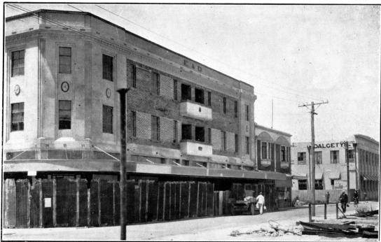
More restoration at the corner of Emerson and Dalton Streets.
