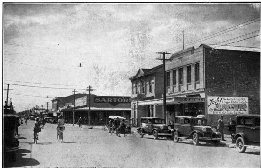
Restored north side of first and second blocks, Heretaunga Street West.
