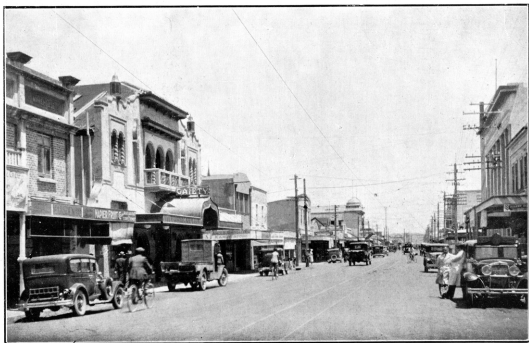
Business back to normal. The reconstructed picture theatre on left.
