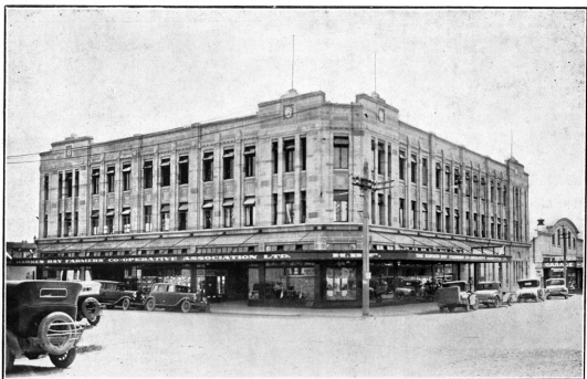
Built to withstand earthquakes, and did so. The Hawke's Bay Farmers' block and garage, Market Street.
