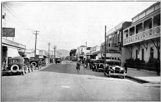
Restoration in 2nd and 3rd blocks, Heretaunga Street East.
