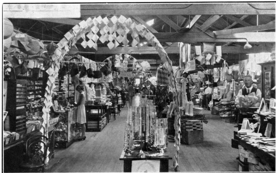
Westerman's temporary premises built since the earthquake, 330 feet long. The premises run from Heretaunga Street to Eastbourne Street.
