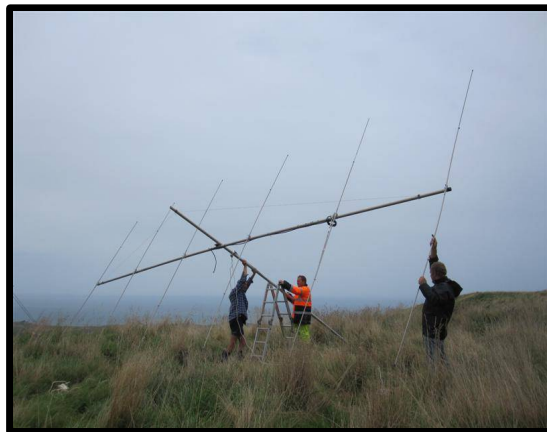
Ready for the erection
