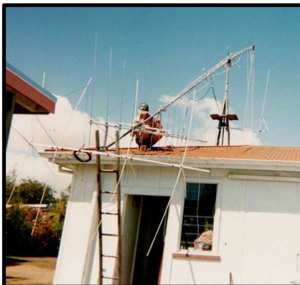
Fitting the four element Quad
