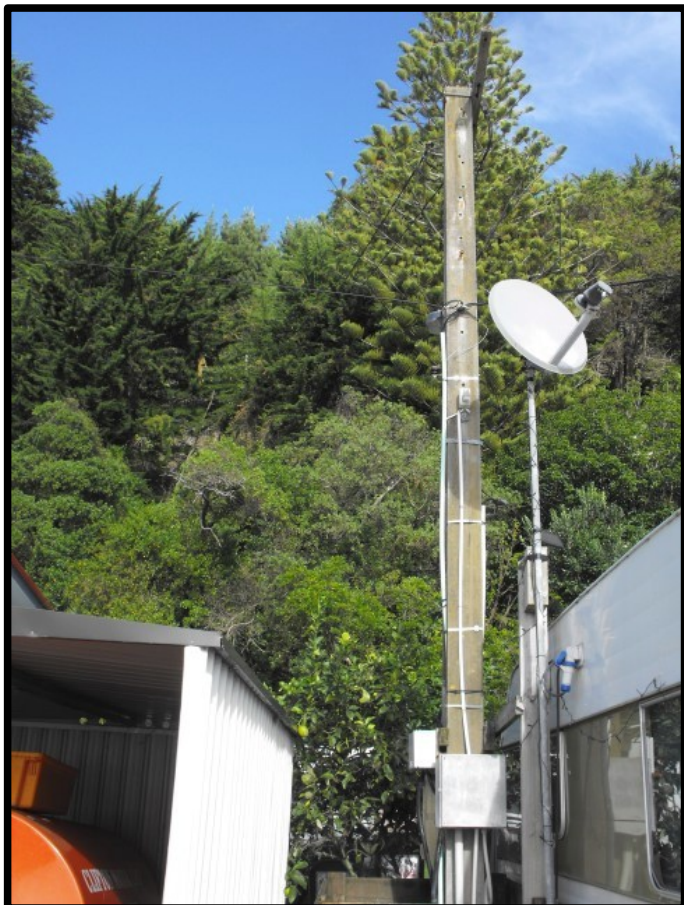
Before (upper pair of wires)
