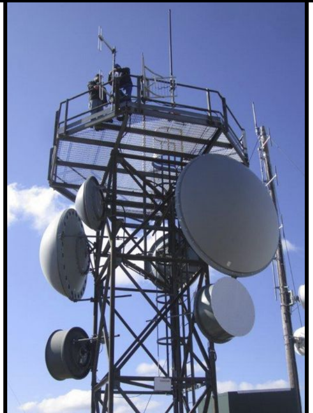
Aerial repairs under way
