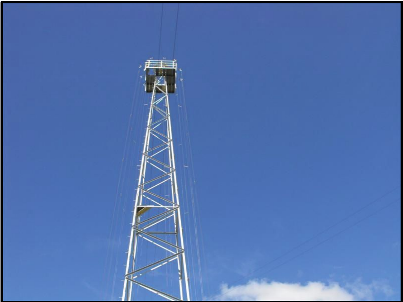
The centre point of the HF receive "Daisy Vee" array, with 620 ft legs and 12 Vee's
