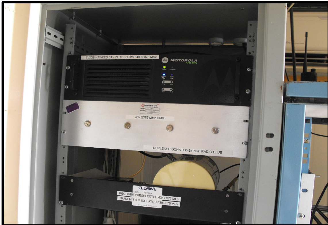
HB UHF DMR Repeater equipment at Mt Threave
