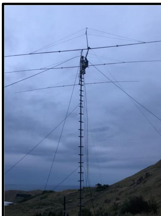
Figure 6: Dec-2019, Alex-DL5LED installing the 3 element 40 m yagi in the last daylight
