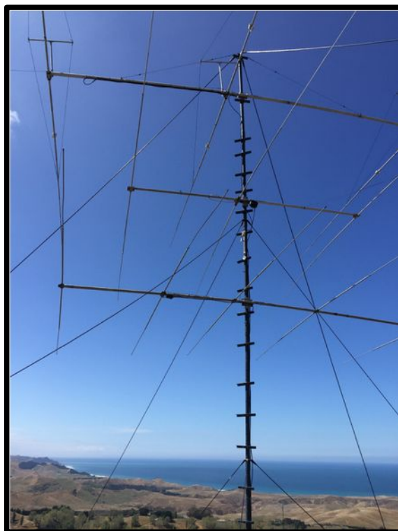
Figure 1: March - 2021, Old airport tower with 3L40m, 3L20m & 5L15m Yagi's installed
