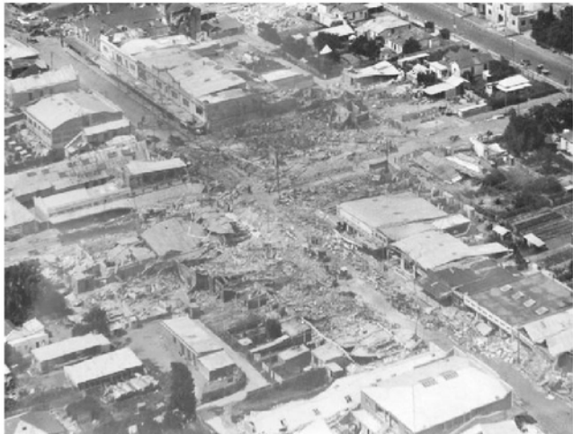
The King Street and Heretaunga Street Intersection after the earthquake.
