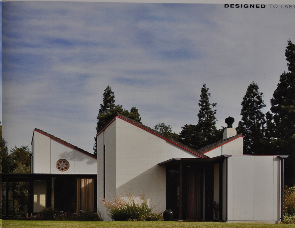
PREVIOUS PAGES, LEFT: Front (northwest) elevation of the Martin House. PREVIOUS PAGES, RIGHT: Window detail, living / dining wing. ABOVE: Full front elevation. From the left: children's wing; covered walkway; dining / kitchen wing; parents' bedroom; roof and chimney above the sitting room.
