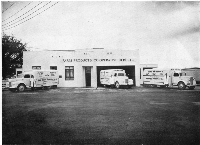
PREMISES (Front View), FARM PRODUCTS CO-OPERATIVE, HAWKE'S BAY LIMITED, HASTINGS.
