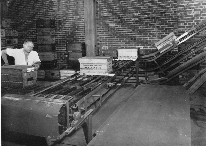
Labour-saving roller conveyors give two-way delivery of egg crates at Combined Co-operative Distributors Limited Egg Packing Station, Christchurch.
