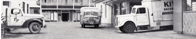
Premises of Farm Products Co-operative (Gisborne), Ltd., Gisborne.
