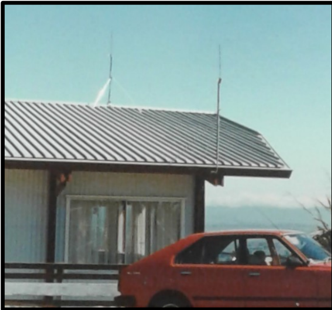
Building roof mounted aerials (1984)
