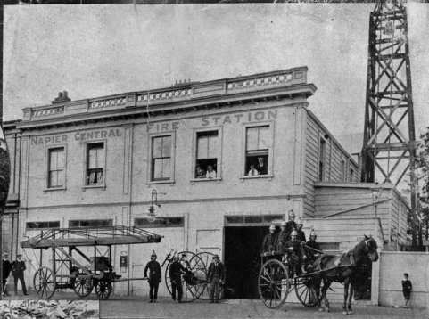
Fire Brigade Station, Herschell St.
