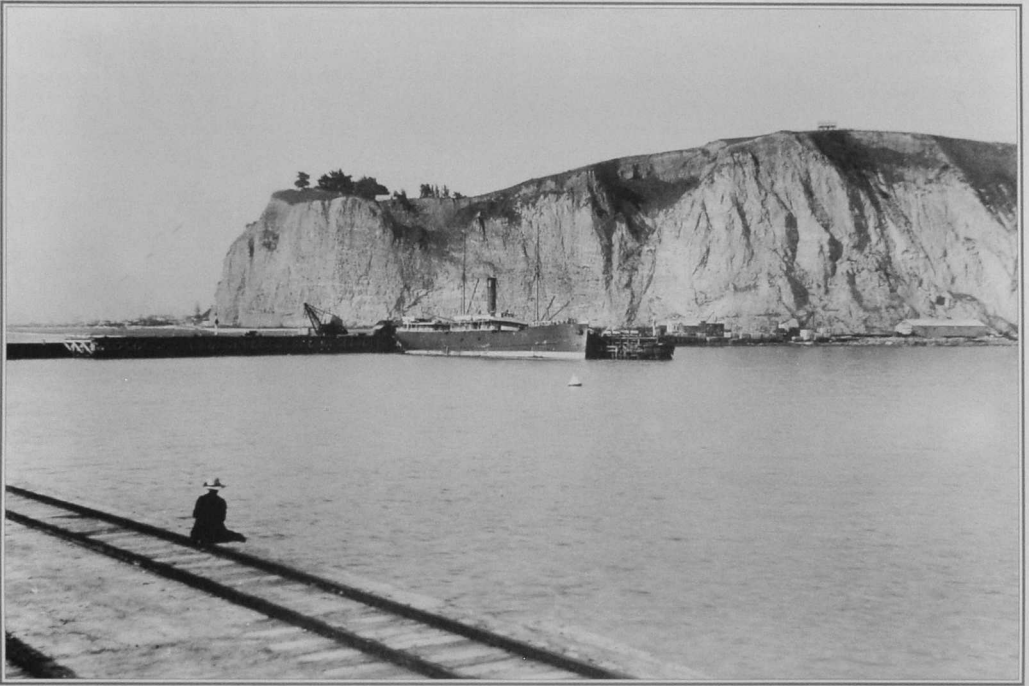
Ship at Claspaw wharf - present breakwater in foreground - 1960.
