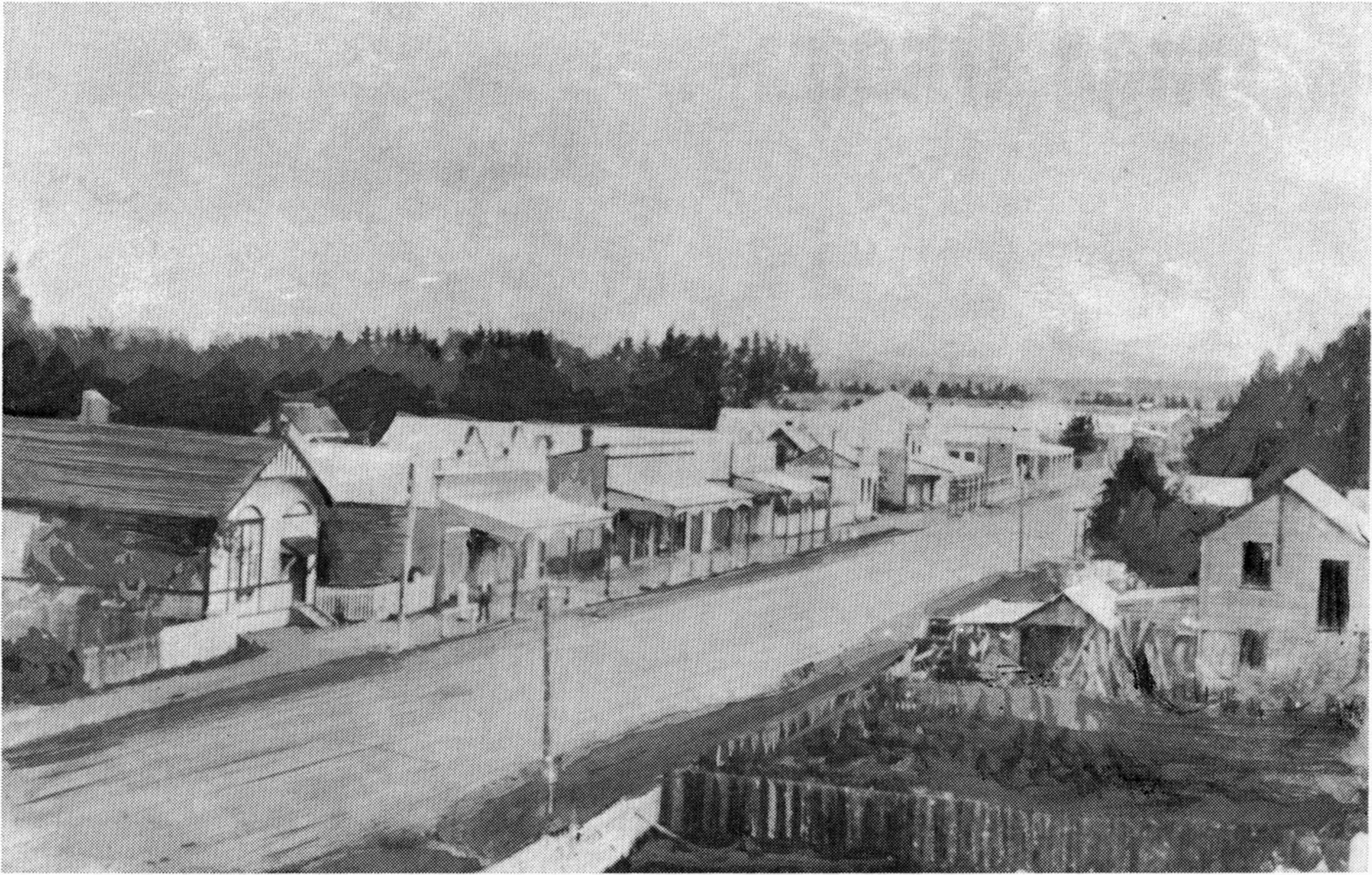
Main Street, Onga Onga, 1913, looking west
