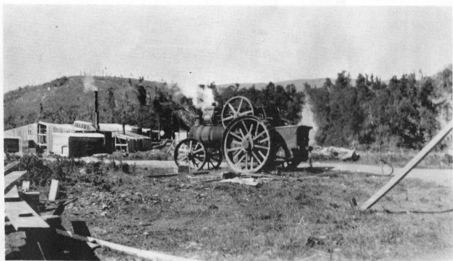
Traction engine at McCullough's Mill. Used for hauling logs & timber. Photo by courtesy of Mrs W. Macdonald.
