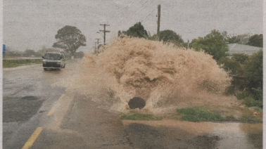
Overflowing stormwater at Haumoana.
