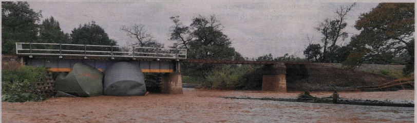
Water tanks jammed under the rail bridge in Harker St, Waipawa.
